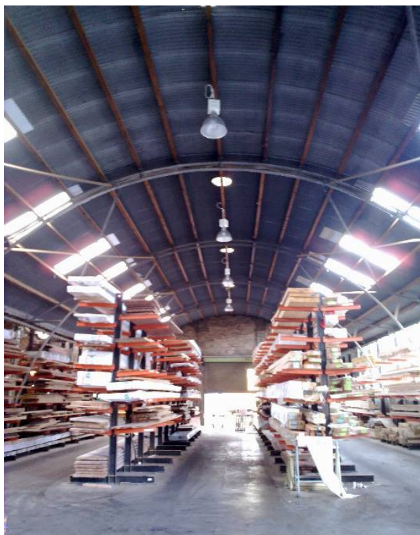
Figure 2: New skylights, vents & lights over DGI warehouse
