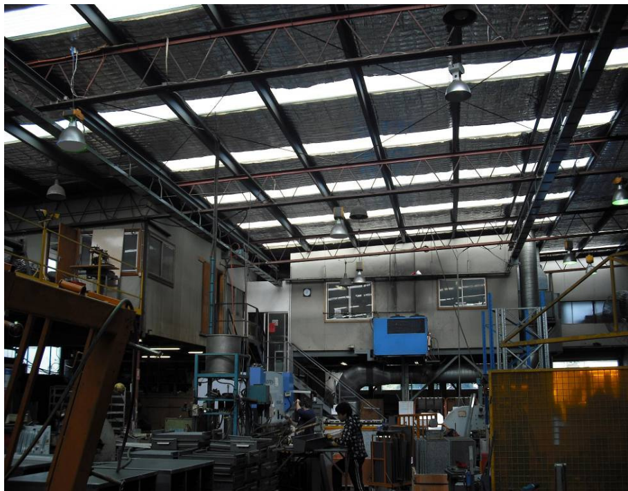
Figure 2: New skylight roofing in the workshop
